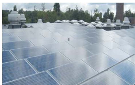
Leicester Primary School – 110.88 kW PV system
